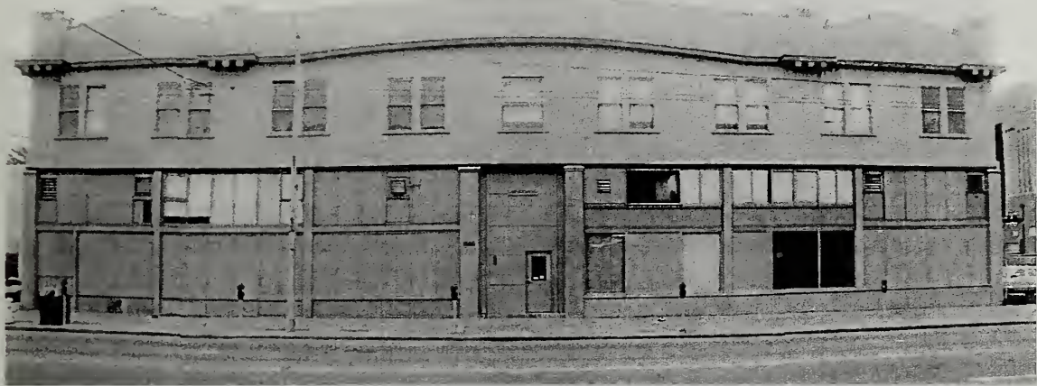
a. Mission Street, Front (East) Elevation
